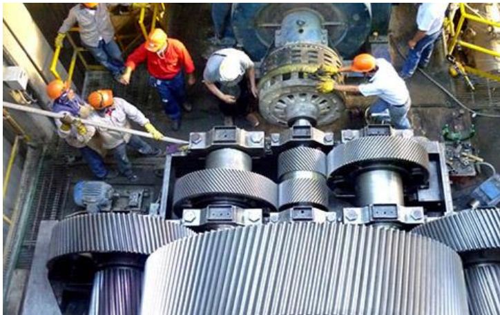
Maintenance of gearboxes
